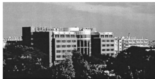
Fig. 19. Smart base isolated building using variable-orifice dampers at Keio University
