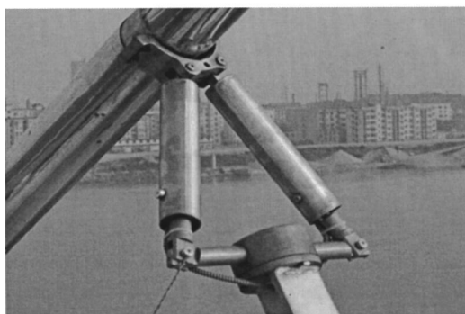
Fig. 18. MR damper installation on the Dongting Lake Bridge, Hunan, China
